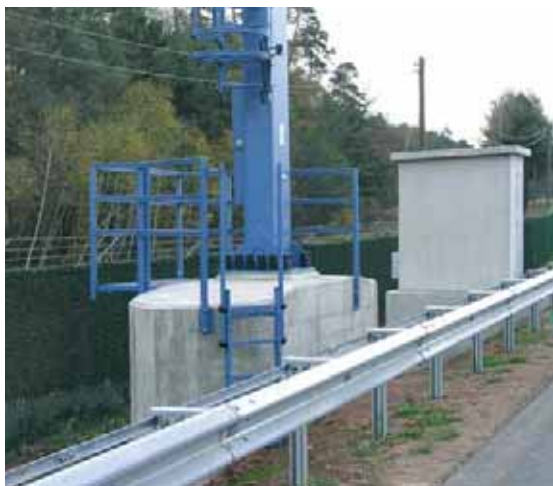
The foundations for the gantries were part of the contract.
