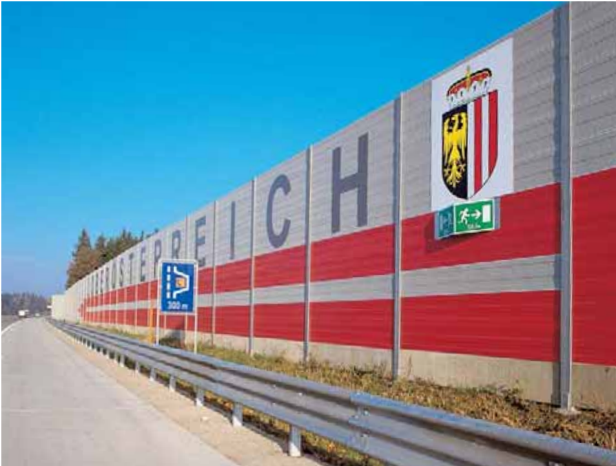
The inscription (the local name for Upper Austria) consists of black metal letters of a height of 2 metres. The coat of arms was digitally printed.
