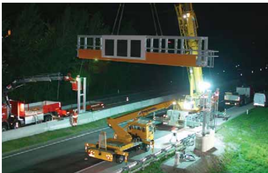
Installing the gantries took a hundred nights.
