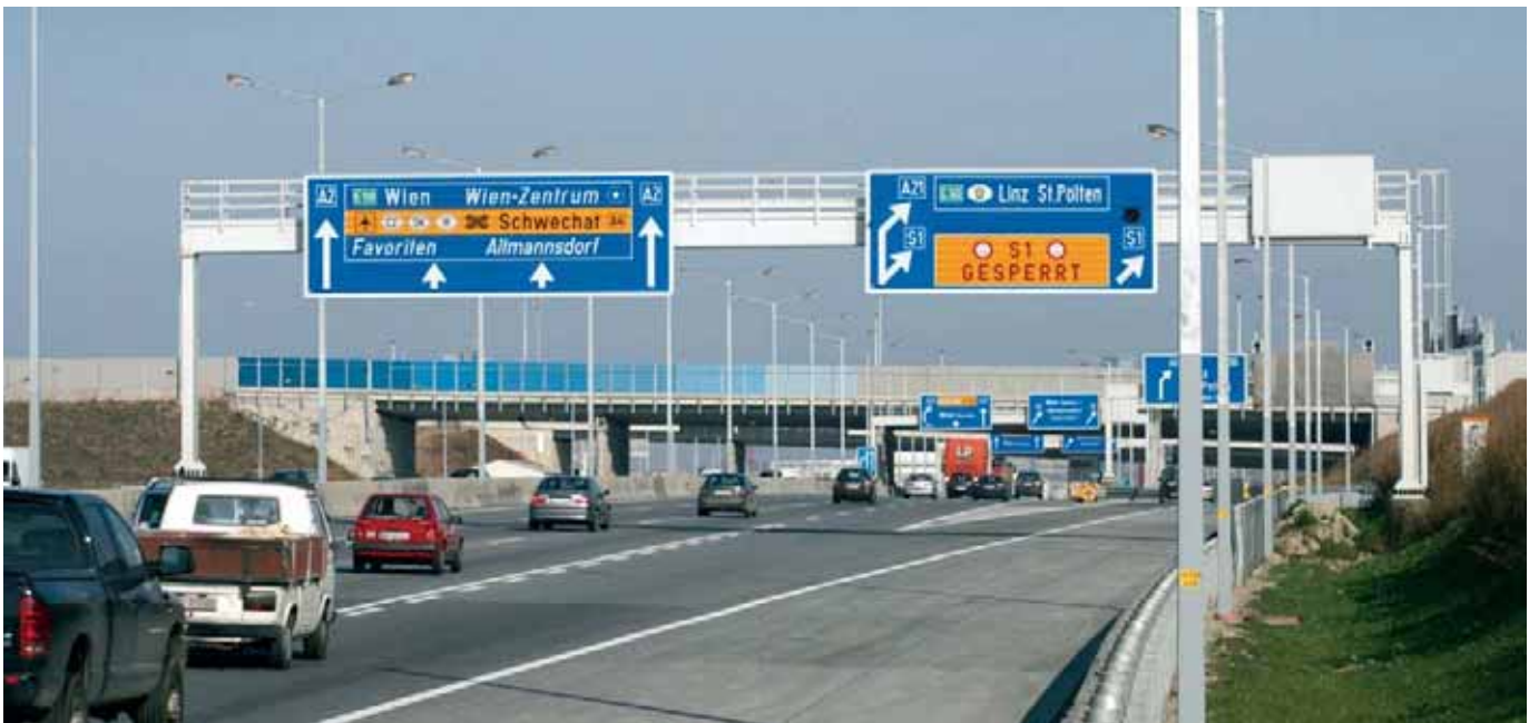
Some 1000 m 2 of type 3 DG sheeting and antidew overlay film were applied to the overhead signs.
